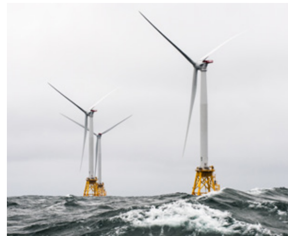
Photo by Dennis Schroeder, National Renewable Energy Laboratory 40389
