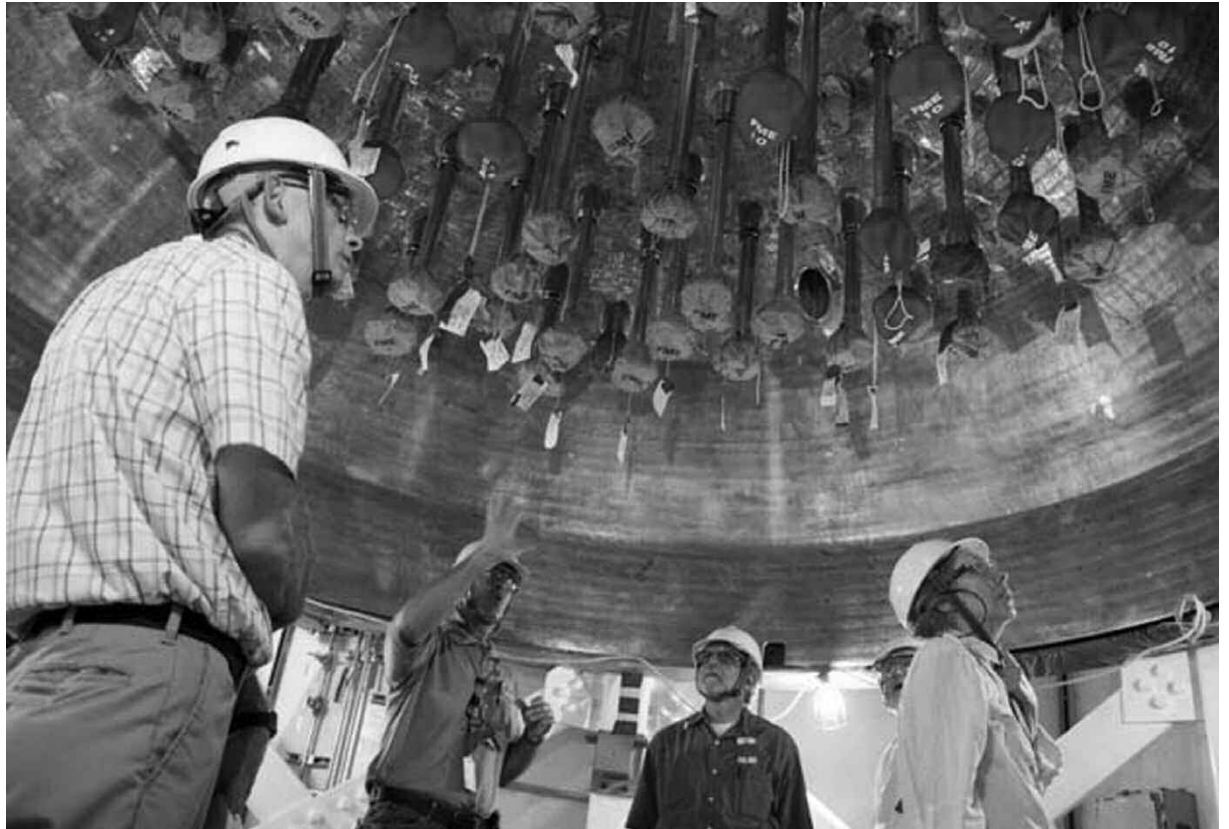
From left: 2 TVA officials, Don Safer, Brian Paddock, and Gretel Johnston from Scottsboro, Alabama. In the reactor core before they lowered the top and well before fuel was loaded
