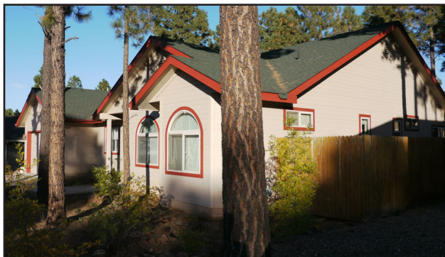
The McCarthy home stays cool in summer and warm in winter due to added insulation. Photo by Jim McCarthy.
