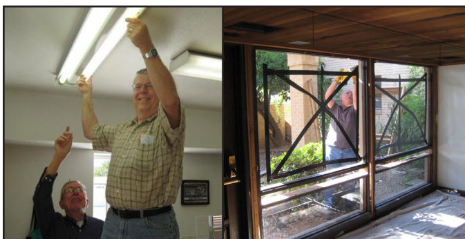
Installing new lights and windows. Photos by Doug Bland.
