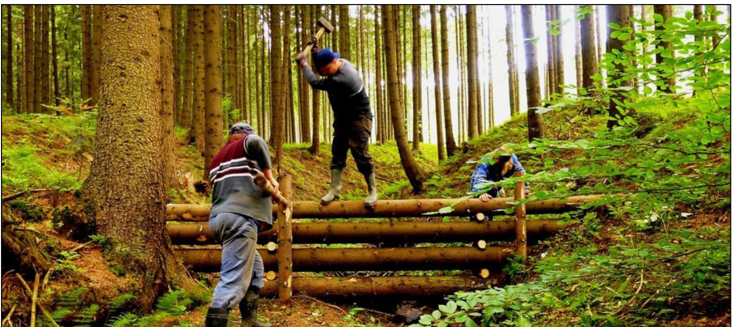
CONTROLLING STORMWATER EROSION IN SLOVAKIA WITH PERMEABLE LOG INTERVENTIONS, A PROJECT OF PEOPLE AND WATER NGO
